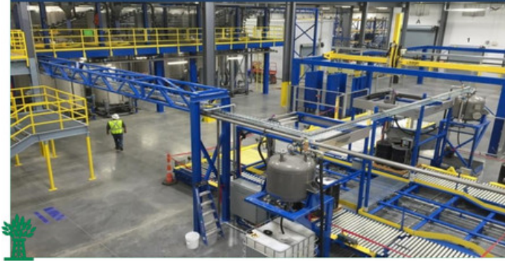
Fluids: Manufacturing Facility & Distribution Center Completed 2016
